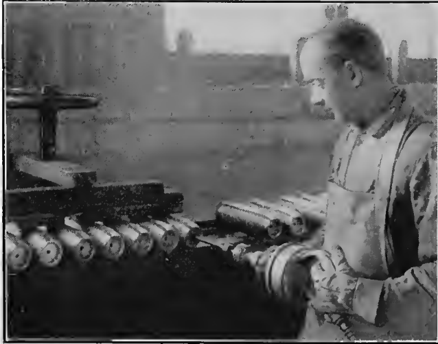
FIG. 23. REAMING THE POWDER TUBES
